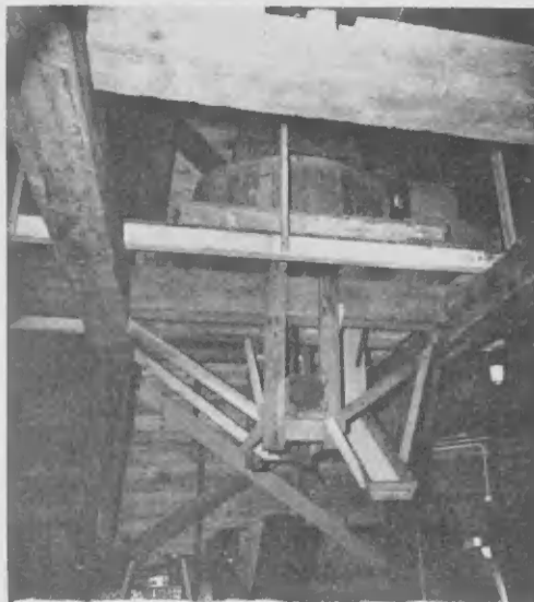
THE FLOUR-grinding mechanism was installed in the mill in 1897. The old Dutch mill, now an Aruba tourist attraction and restaurant, was built in 1815. E MECANISMO di mola harinja a worde instala den e mulina na 1897. E mulina Holandes bieuw, awor un atraccion pa turista, a worde traha na 1815.
